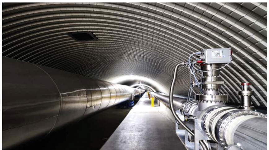
Figure 5. View inside the Virgo tunnel showing the filter cavity vacuum pipe running alongside the north arm of the interferometer.
